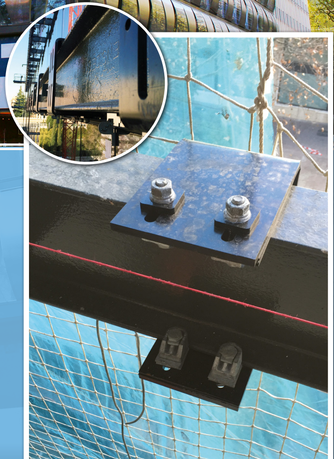
Type AF girder clamps connect the C-shaped brackets to the steel sections of the main building structure
