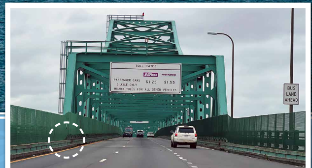
The bridge required upgrades to improve traffic management and safer work zones
