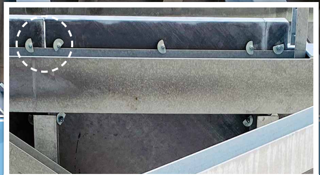
FloorFast installed underneath the finished floor
