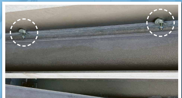
FloorFast stepped cast body securely clamps to the steelwork
