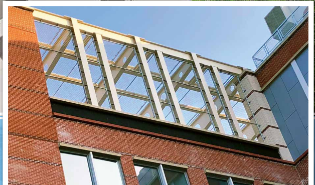
The completed steel framed rooftop enclosure
