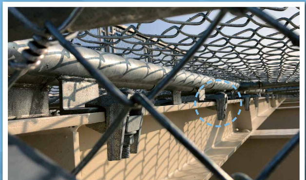
Type F3 flange clamp connect the mesh panels
