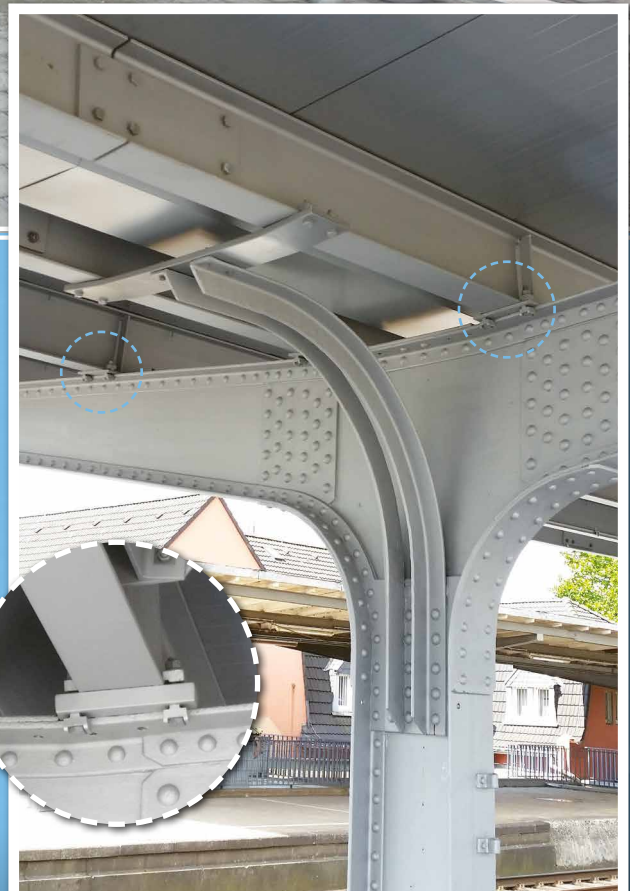
Steel beams are connected to the columns
