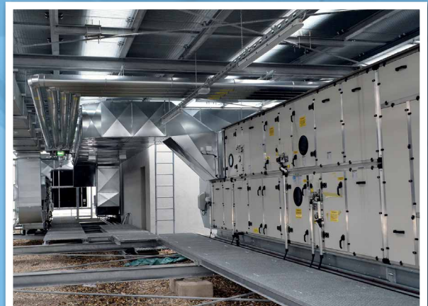
Steel beams create the extra floor
