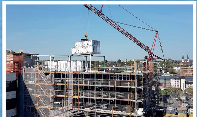
Air conditioning units being installed
