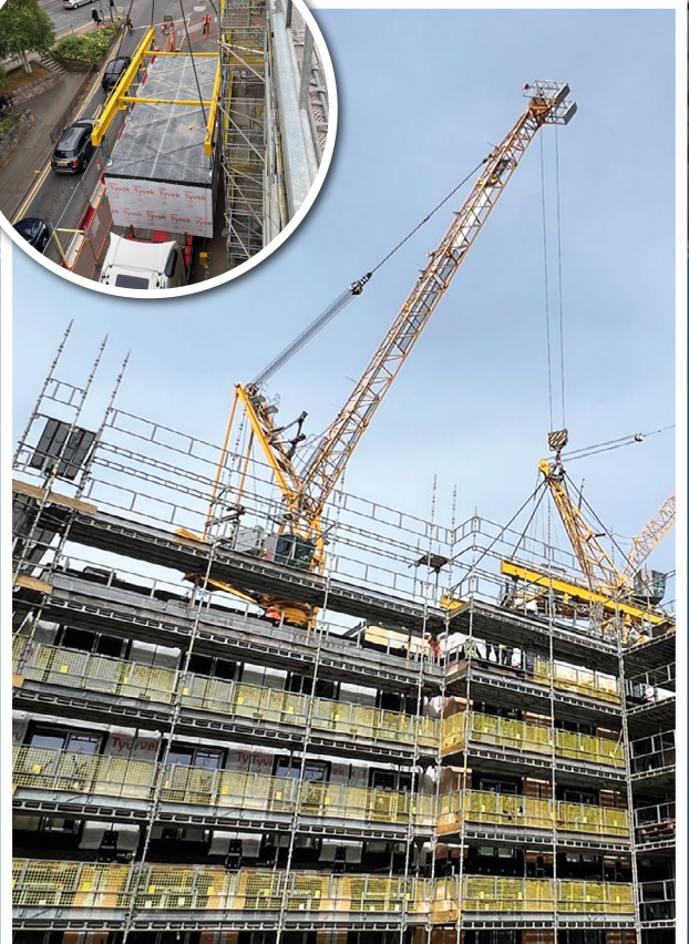
Modular units carefully stacked on top of each other
