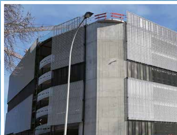
The completed cladding system
