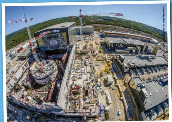
ITER nuclear facility under construction
