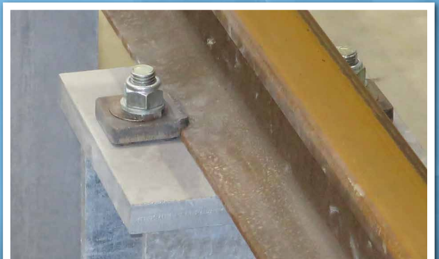
Type HD rail clips used to secure the rails
