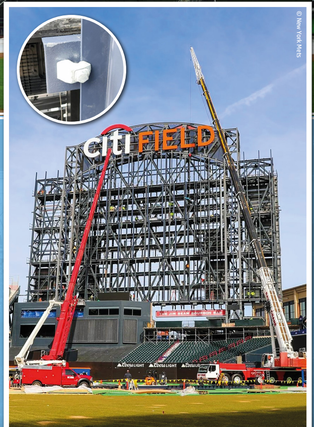
Type AAFs connect the angle brackets to the steel columns
