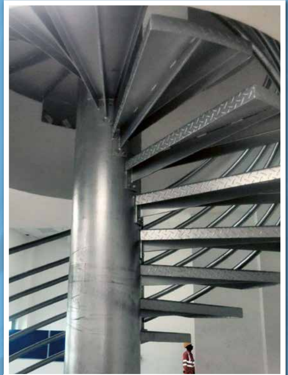
Installation was required from one side only
