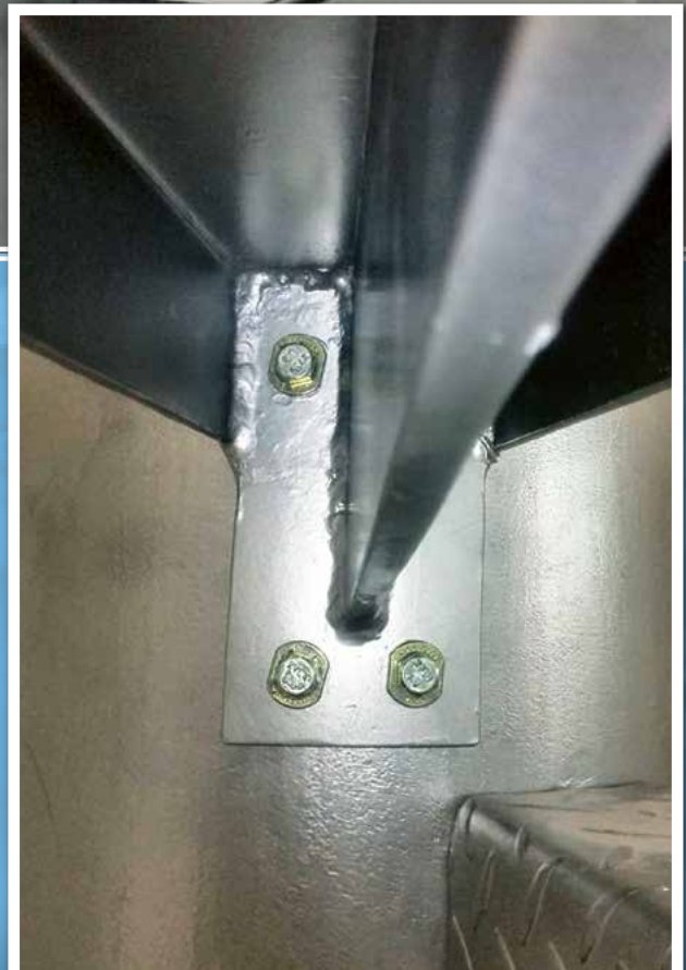
Hollo-Bolts were inserted into pre-drilled holes
